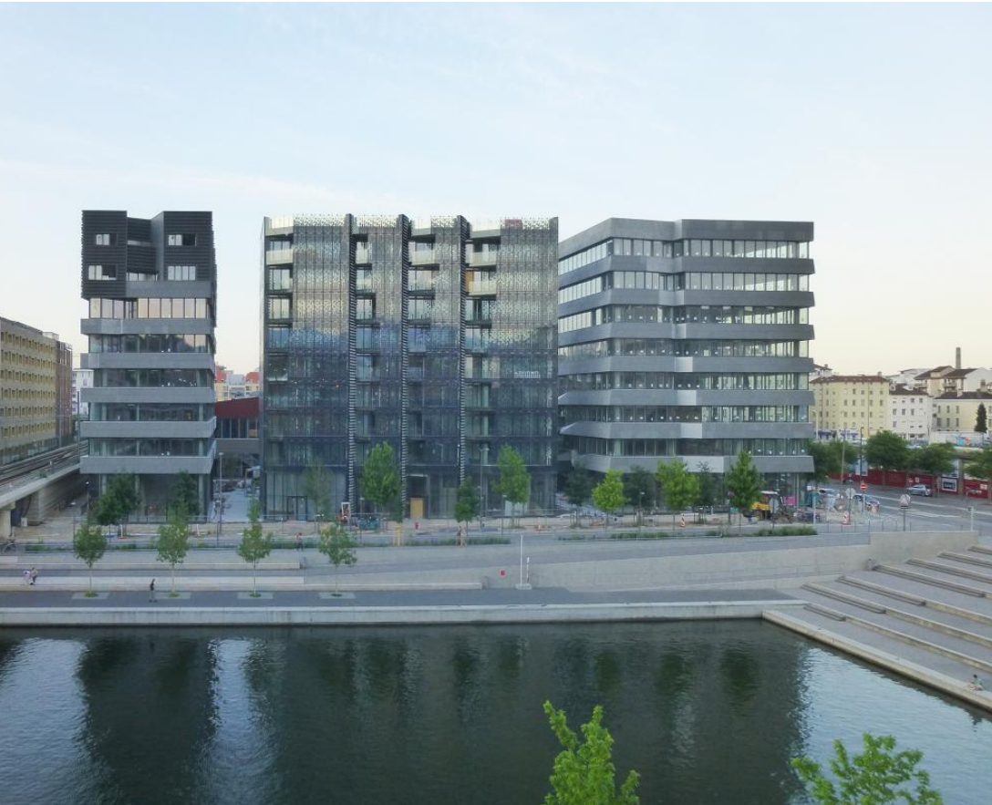
Lyon, Confluence, 2014 HIKARI Kengo Kuma and Associates Forrás: https://www.tess.fr/en/projet/hikari-building
